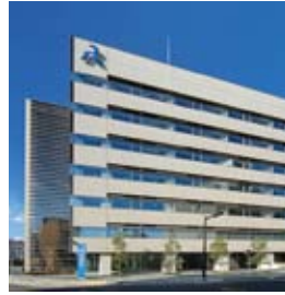
Chuo Labour Bank Operating Center (Yokohama-city, Kanagawa)
