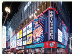
Nakaza Kuidaore Bldg. (managed property)
