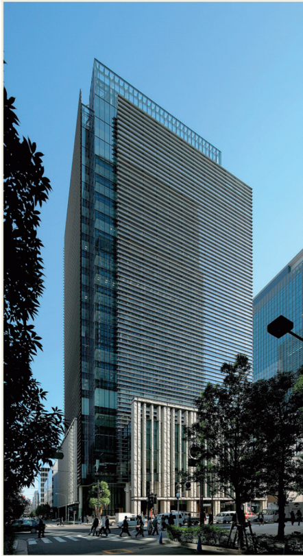
Nihombashi Muromachi Nomura Building
