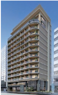
Hotels Began construction on the tentatively named NOHGA HOTEL Shinjuku Gyoen, slated to open in 2027
