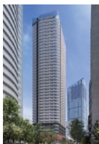
Atago District Category 1 Urban Redevelopment Project F District
