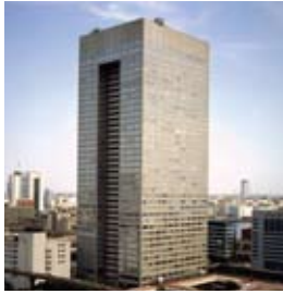
Toshiba Building (Minato-ku, Tokyo)
