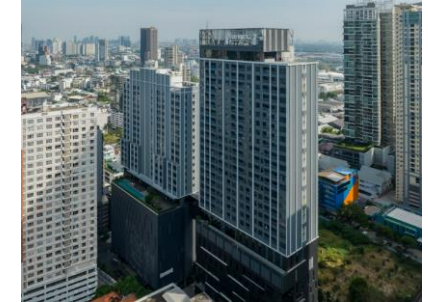
Staybridge Suites Sukhumvit (Bangkok) Completion: 2023 Major use: Service apartment Total units: 411
