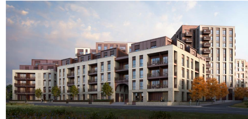
Herne Hill Project (London) Completion: 2028- (Planned) Major use: Rental housing Total units: 218
