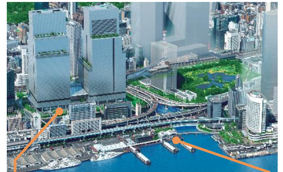
Taking advantage of its location connecting land, sea, and sky to become Tokyo's new water transportation hub
