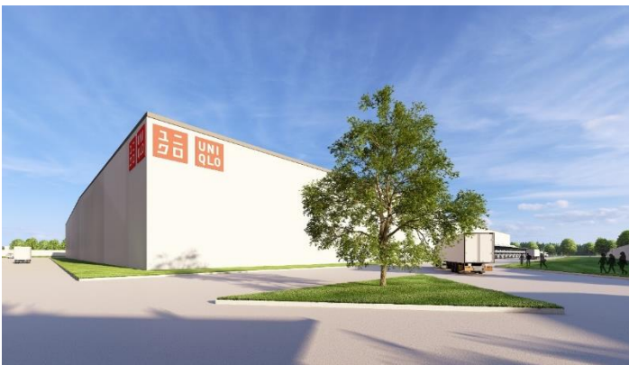
Cavite project, logistics facility * (Cavite, the Philippines/started the construction in June 2024)
