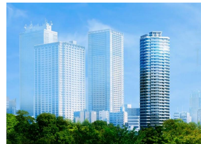
PROUD TOWER Higashi-Ikebukuro Station Arena
