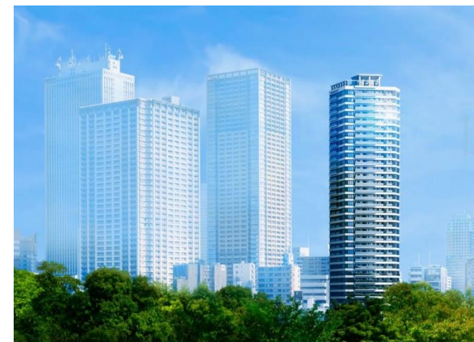
PROUD TOWER Higashi-Ikebukuro Station Arena
