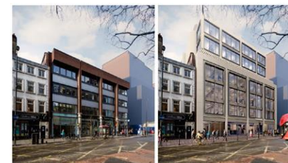
Current state After refurbishment
