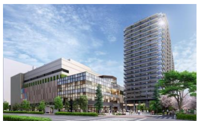
・(tentative name)Kagurazaka Fukuromachi Project ・(tentative name)Musashiurawa station front Project
