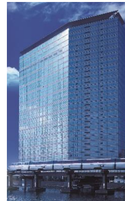
Nomura Fudosan Tennozu Building
