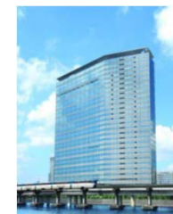
Nomura Fudosan Tennozu Building
