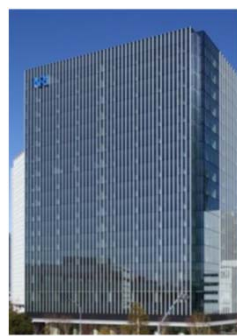
Yokohama Nomura Building
