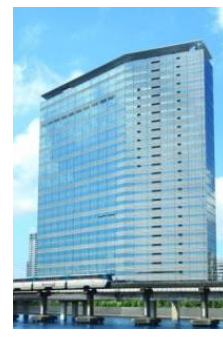
Nomura Fudosan Tennozu Building
