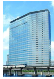
Nomura Fudosan Tennozu Building
