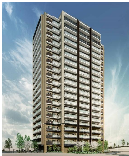
PROUD Tower Higashiikebukuro
