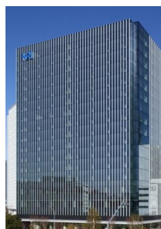
Yokohama Nomura Building
