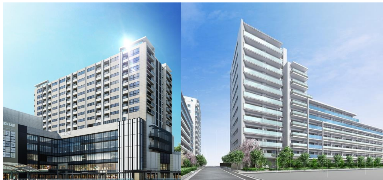
PROUD Fuchu Station Arena
