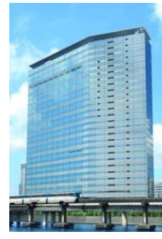
Nomura Fudosan Tennozu Building
