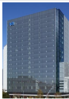
Yokohama Nomura Building
