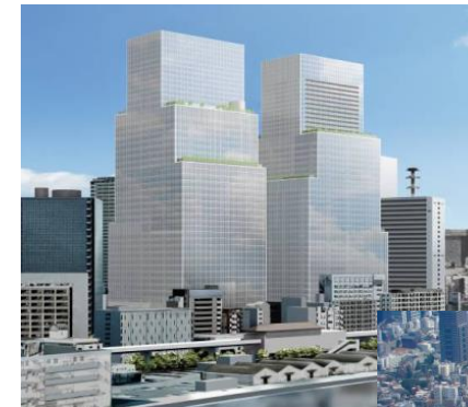
Shibaura 1-chome rebuilding
