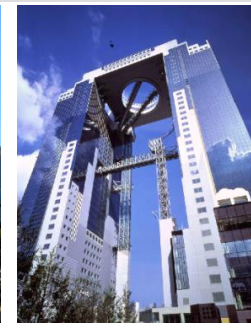
Umeda Sky Building
