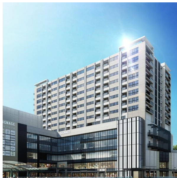
PROUD Fuchu Station Arena
