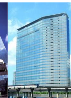
Nomura Fudosan Tennozu Building
