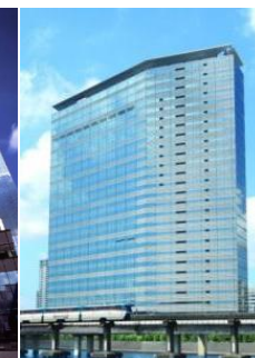
Nomura Fudosan Tennozu Building
