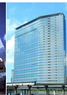
Nomura Fudosan Tennozu Building
