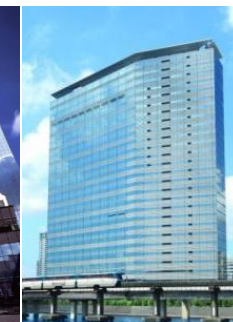
Nomura Fudosan Tennozu Building
