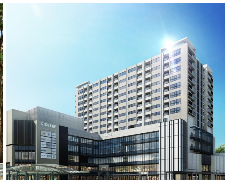
PROUD Fuchu Station Arena
