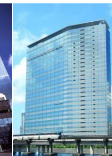
Nomura Fudosan Tennozu Building
