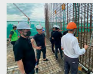
On-site construction check (Vietnam)
