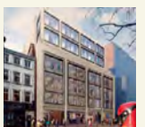
The image of building after renovation
