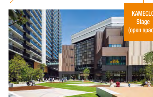
An open space is available for use by visitors and residents. It provides a place for local residents to interact.
