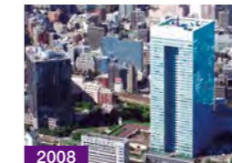
2008 NREG TOSHIBA BUILDING joined the Group
