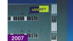
2007 Completed construction of Landport Atsugi
