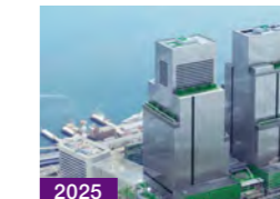
2025 Started construction of Shibaura Project (South Tower)
