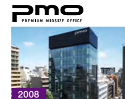
2008 Completed construction of PMO Nihonbashi Honcho
